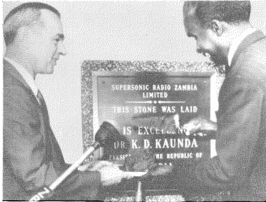
Figure 3—His Excellency Dr. Kenneth Kaunda, President of the Republic of Zambia, and Rex B. Grey, Chairman of Standard Telephones and Cables and of Supersonic Radio Zambia, at the laying of the foundation stone of the new plant in Livingstone.
